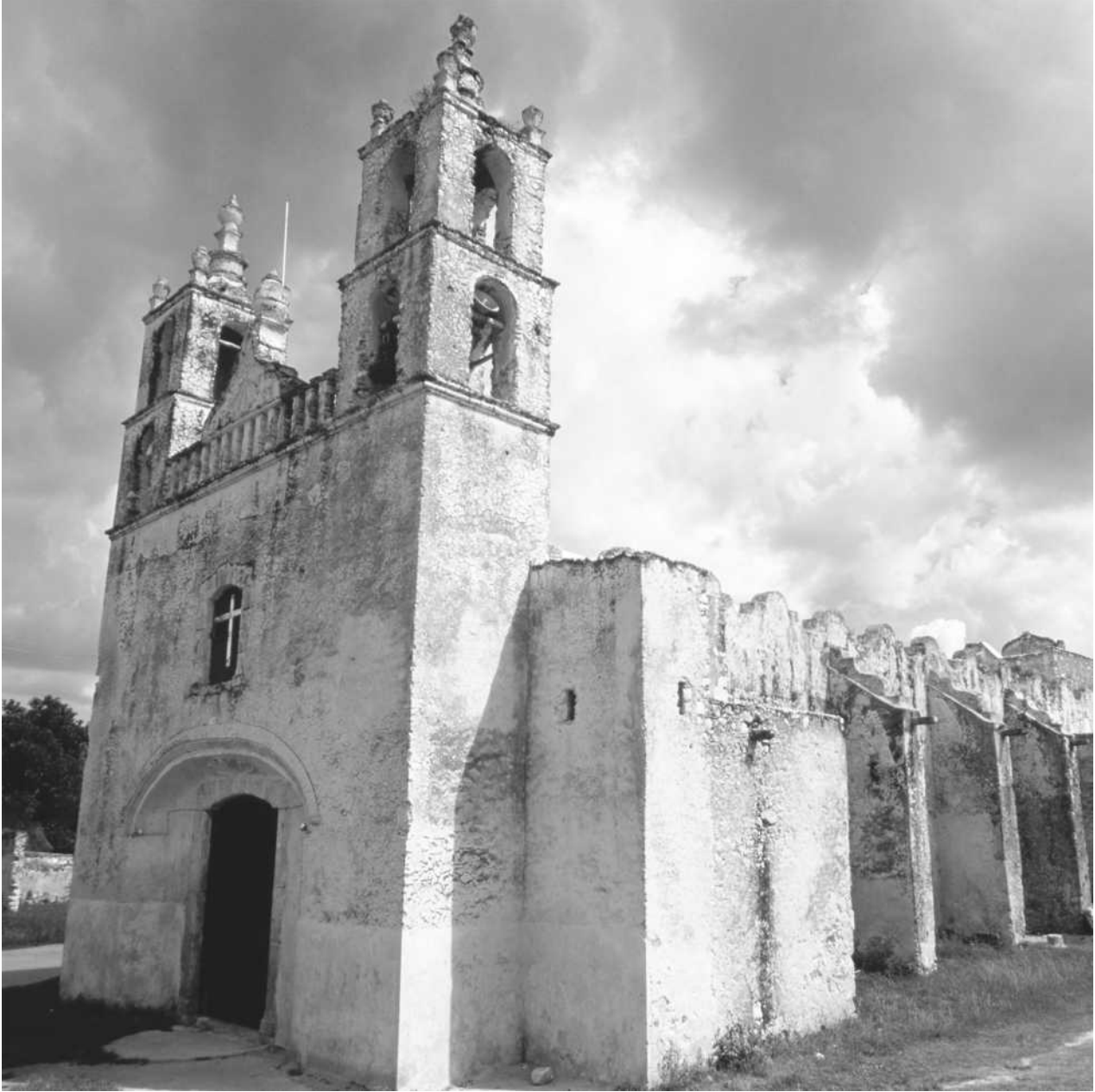
This colonial church with two bell towers was built with ancient Maya stones. Spanish and French architectural traditions influenced Mexican buildings.
